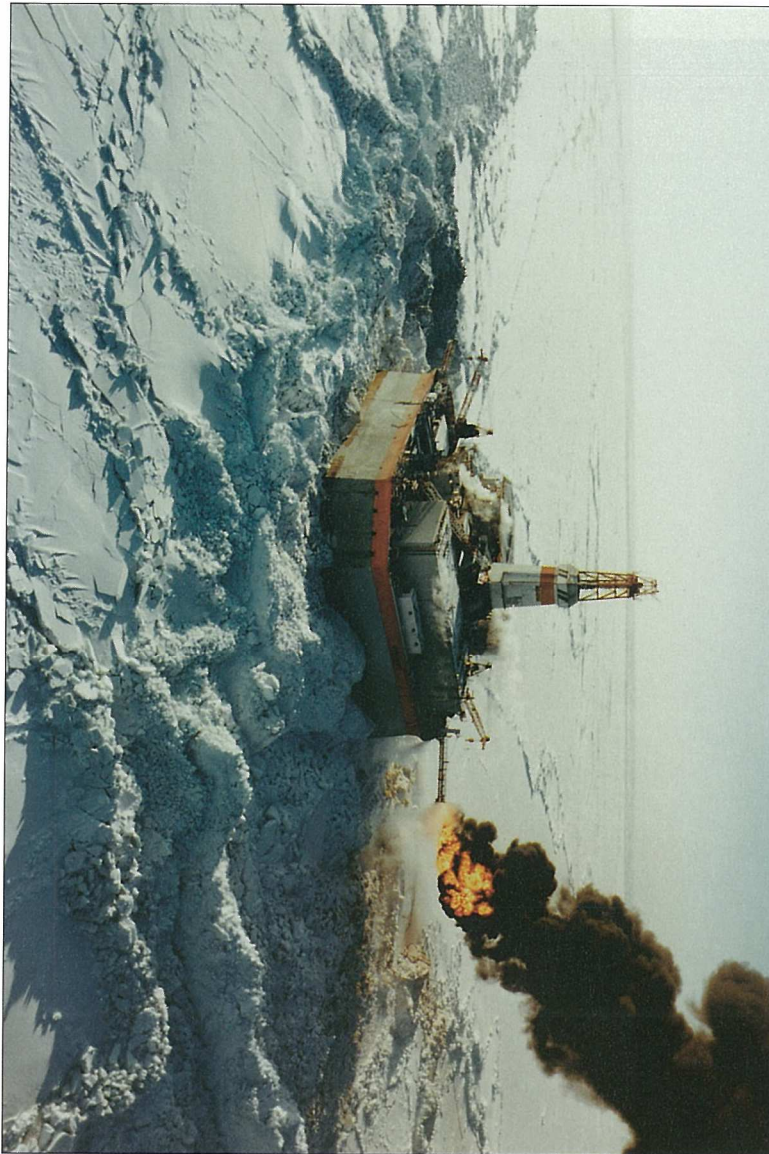
Photograph 2. Molikpaq Platform under ice attack during hydrocarbon exploration drilling in Canadian offshore Arctic (Photo courtesy of Gulf Canada Resources Inc.)
