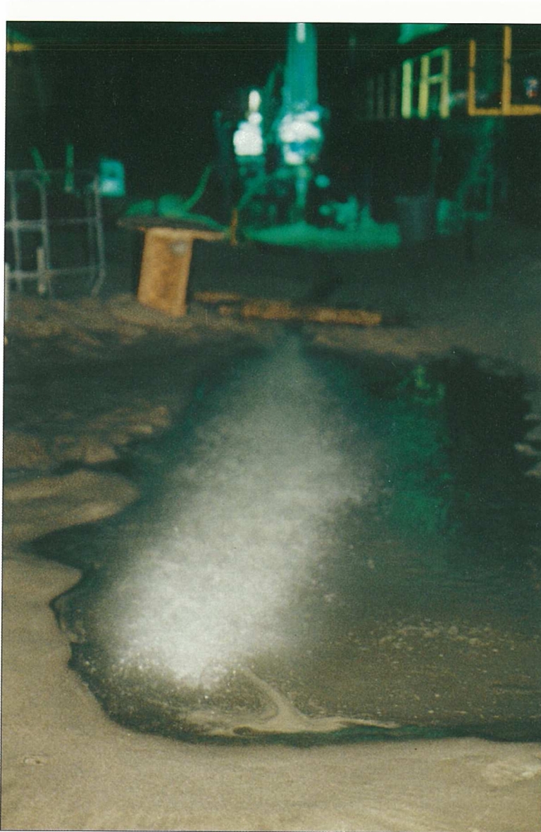
Phototograph 4. Vibro-Drain operating in Molikpaq Core showing water discharge from filter/drain module exhaust
