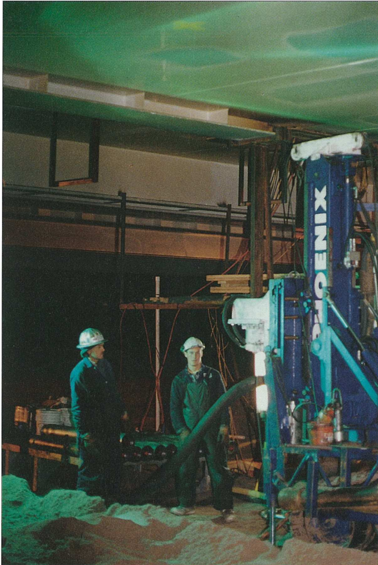
Photograph 3. Vibro-Drain operating in Molikpaq Core showing deployment under restricted headroom
